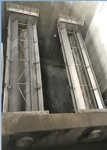
Ortho-Wash™ Troughs with Pipe Outlet
