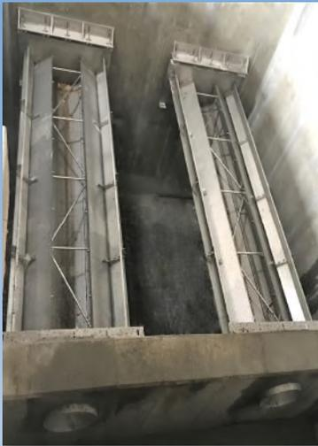
Ortho-Wash™ Troughs with Pipe Outlet
