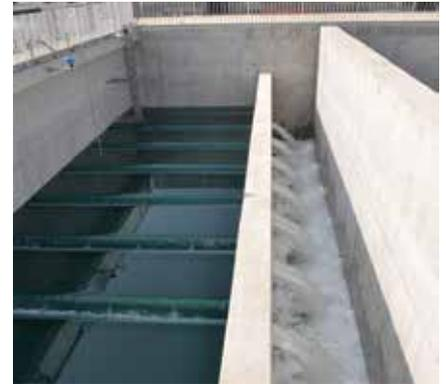
which vary water and air flowrates considerably under different operating conditions. Lateral underdrains are often fixed in place by grout or anchor bolts and buried in gravel to support and retain media and improve backwash performance.
